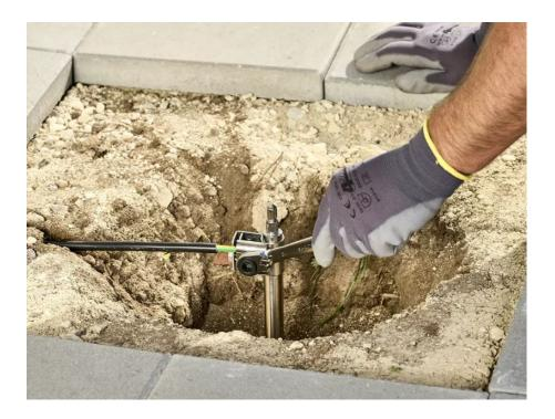
Standardised, efficient and easy to install: The D18014 earth rod set from DEHN for retrofitting earthing systems Photo: DEHN SE
